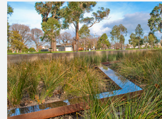
Stormwater treatment raingarden
