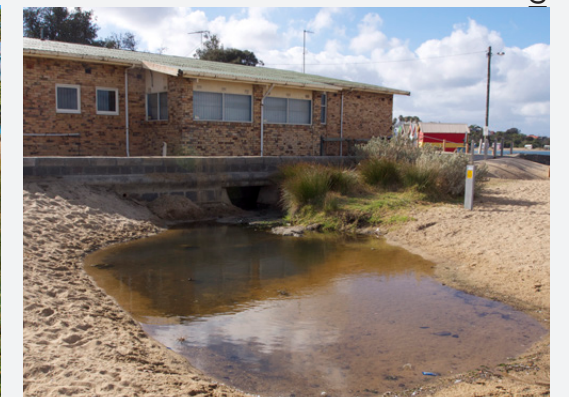
Existing stormwater outfall
